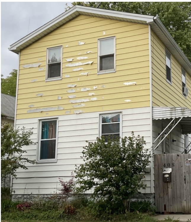
Peeling paint and entrance awning require maintenance, but the home is structurally sound.
