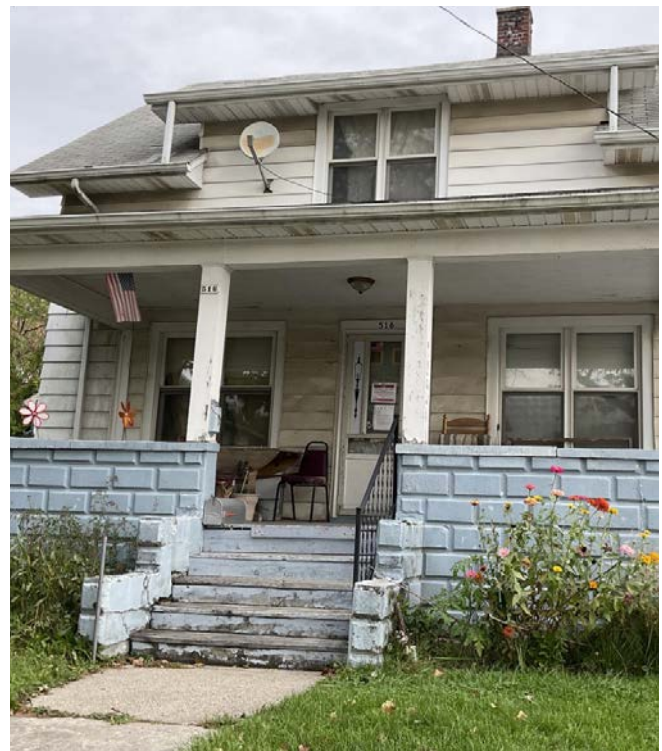
Porch steps may require fresh paint or reinstallation. Discoloration in roof's soffit area requires cleaning or fresh paint.
