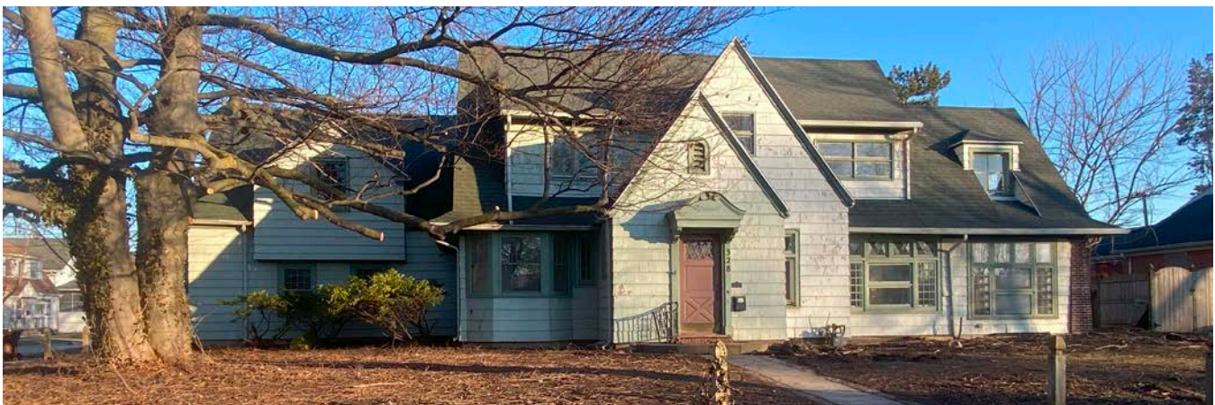
Single-family home in Monroe in the midst of renovation
