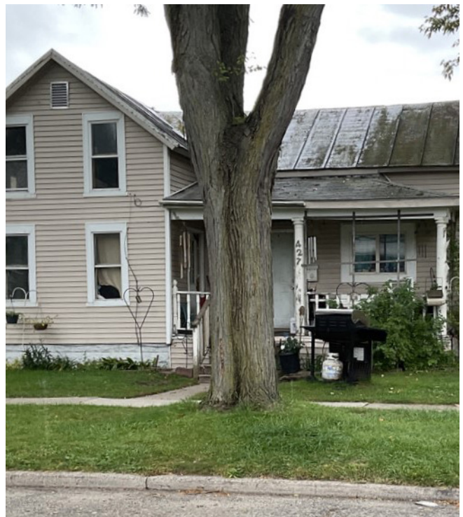
Roof discoloration requires intensive maintenance, and both chimney and porch awning require cleaning. Landscape is marginally maintained.
