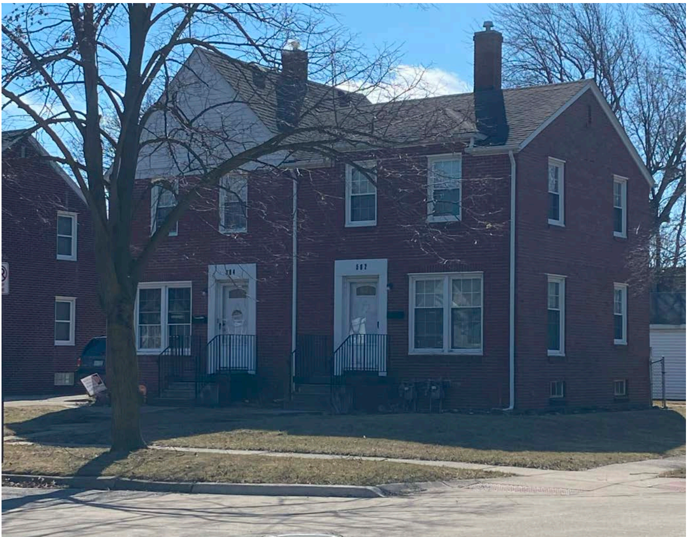
Duplex in Monroe that fits in with the context of the surrounding neighborhood.
