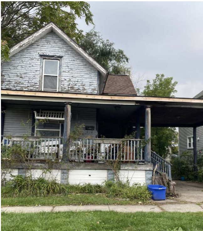
Deteriorating exterior of front façade, front porch, and windowpane require both structural improvements and new paint. Clutter on the porch should be cleared, and front landscaping requires maintenance.
