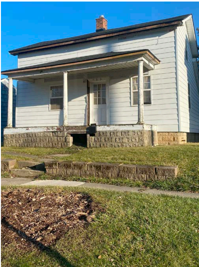
Monroe home in disrepair
